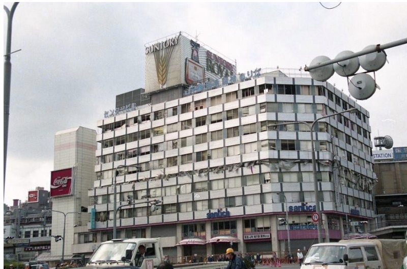
Figure 1 – An astonishing earthquake-induced structural failure found on the surface in Kobe in January 1995. The reinforced concrete (RC) buildings near Sannomiya railway station looked completely safe at first sight, but the middle floor was vertically compressed and it totally disappeared (Photograph courtesy of Kobe City).
