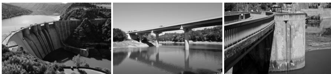
Figure 1 – Example of structures where ASR and DEF are often observed (left and middle) and of the cracking resulting from their development (right)
