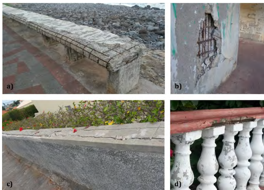
Figure 1 - Degradation of constructions due to reinforcement corrosion: a) seat bank / fence between ocean beach and promenade; b) buttress vault; c) concrete block wall with reinforced mortar at the top; and d) concrete fence
